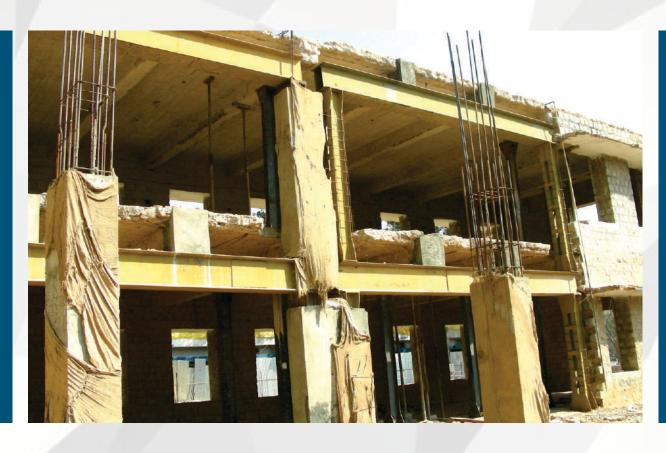
Post-tensioning of Carbon Laminate at Beam bottom
